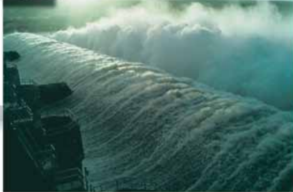
Tucuruí hydroelectric plant - Photo on loan from Eletronorte
