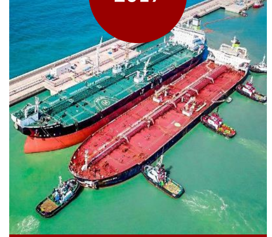
Oil Terminal – Açu Petróleo
